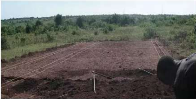
Foundation laying out
