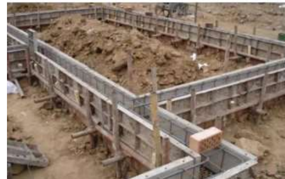
Foundation formwork support
